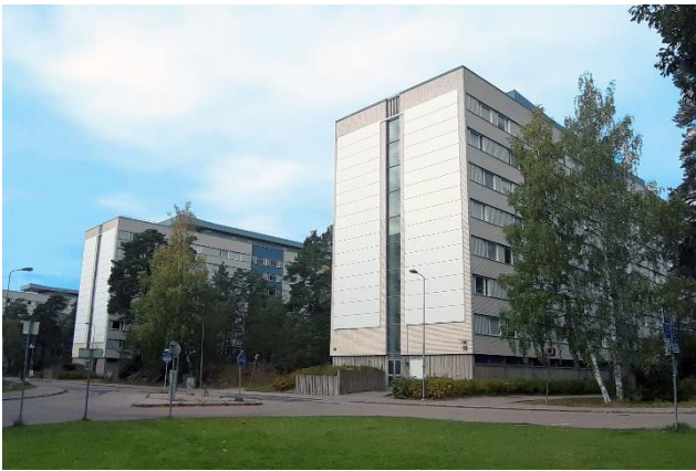
Sun city project Flogsta in Uppsala, Sweden, September 2019
