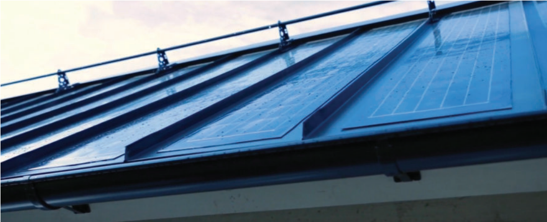
Fig. 2 Detail of the BIPV roof. Source: Midsummer.
