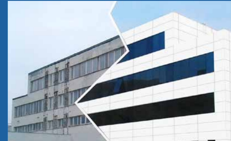
renovated and active
