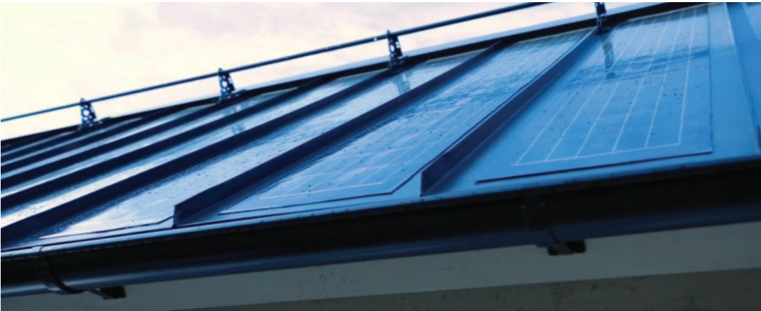
Fig. 2 Detail of the BIPV roof. Source: Midsummer.
